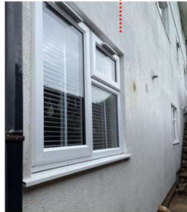
Figure 5 - New window positioned far south on the eastern elevation
